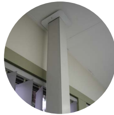
power pole to ceiling
